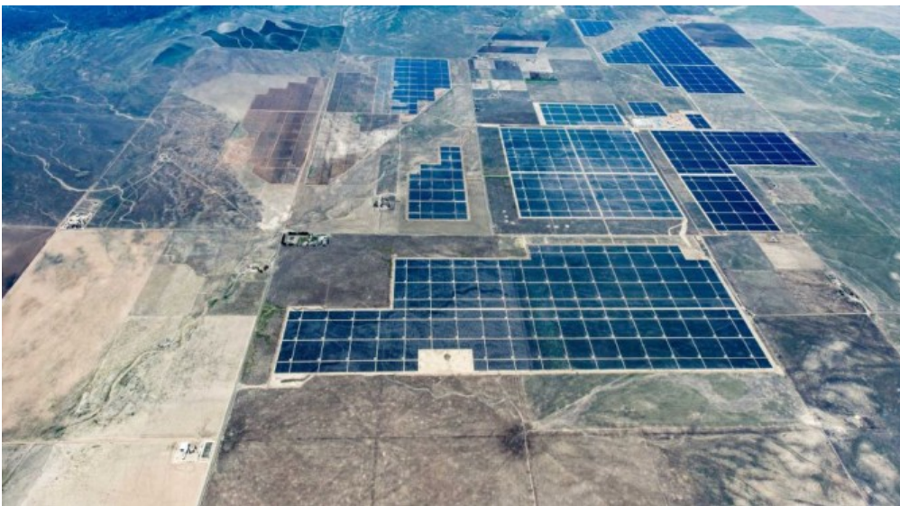
World's largest solar photovoltaic farm – California (500 megawatts, operational in 2014)
