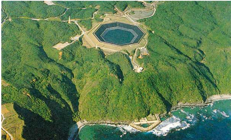
Figure 57. Pilot Seawater Pumped-storage Power Plant, Okinawa Pref. in Japan. The octagonal shape shows the upper dam. The outlet of the tailrace is surrounded by tetra-pods for protection from waves. The picture is from the 1998 Hitachi Review.
