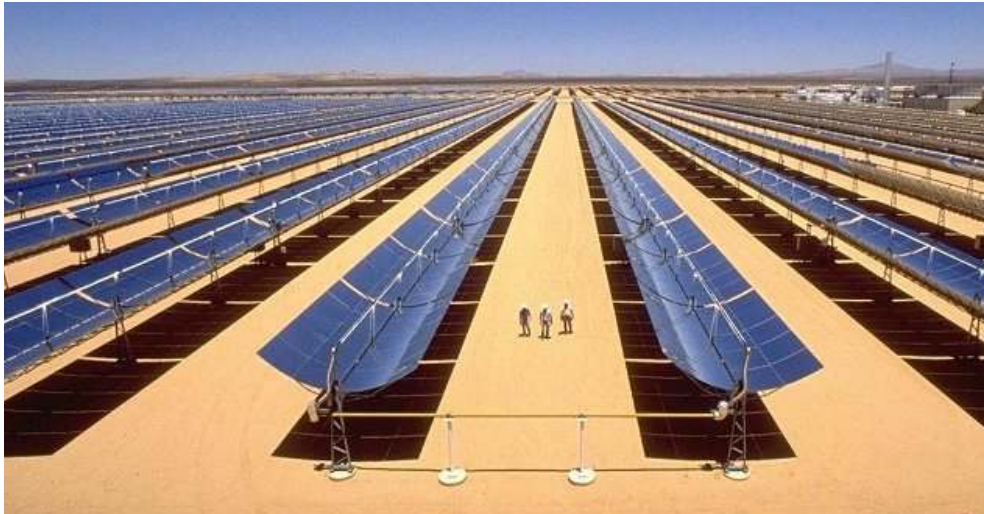
Figure 5. An excellent illustration of why it is difficult to collect sunshine from all the land. At noon only one third of the sunshine hits collectors.
