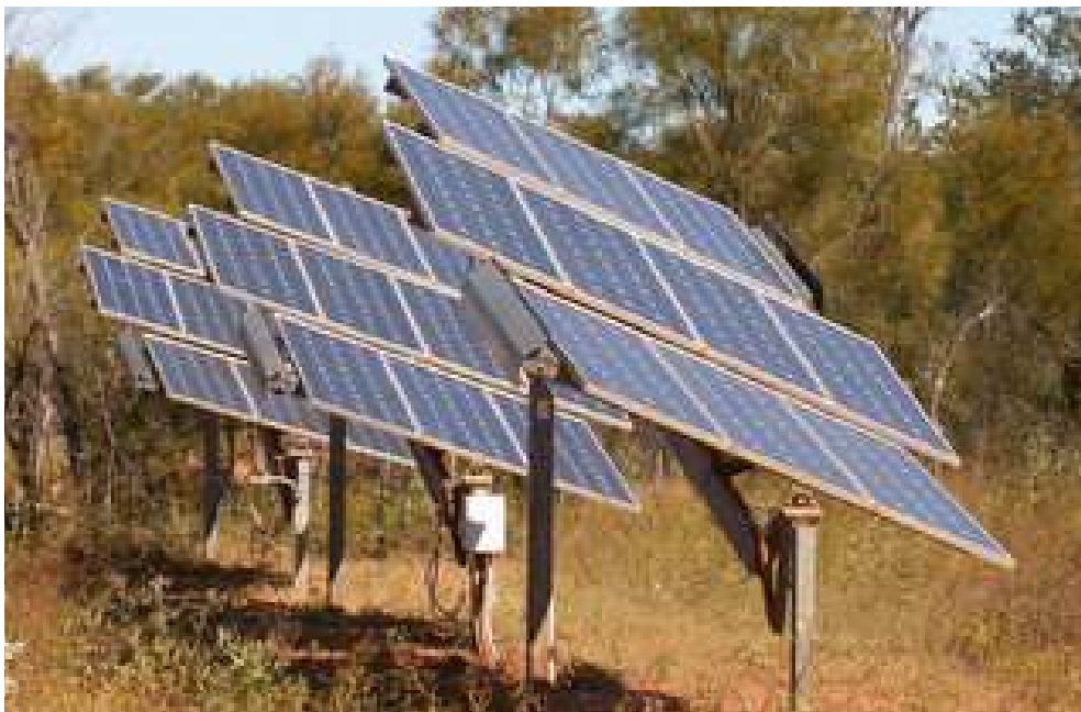
Figure 3. Clever tracking solar array. Cylinders of ammonia on each side of the array are connected by a tube. Shading is arranged so that when the sun hits the cylinder on one side, the fluid boils and passes to the other side where it condenses. The weight tilts the panel until the cylinders are equally shaded. These panels are at Broome at latitude 17^\circ\text{S} .
