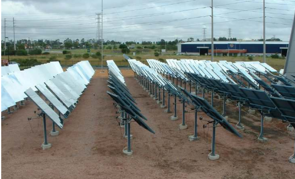
Figure 4. Concentrating solar thermal mirrors similar to those planned for the Cloncurry power station.
