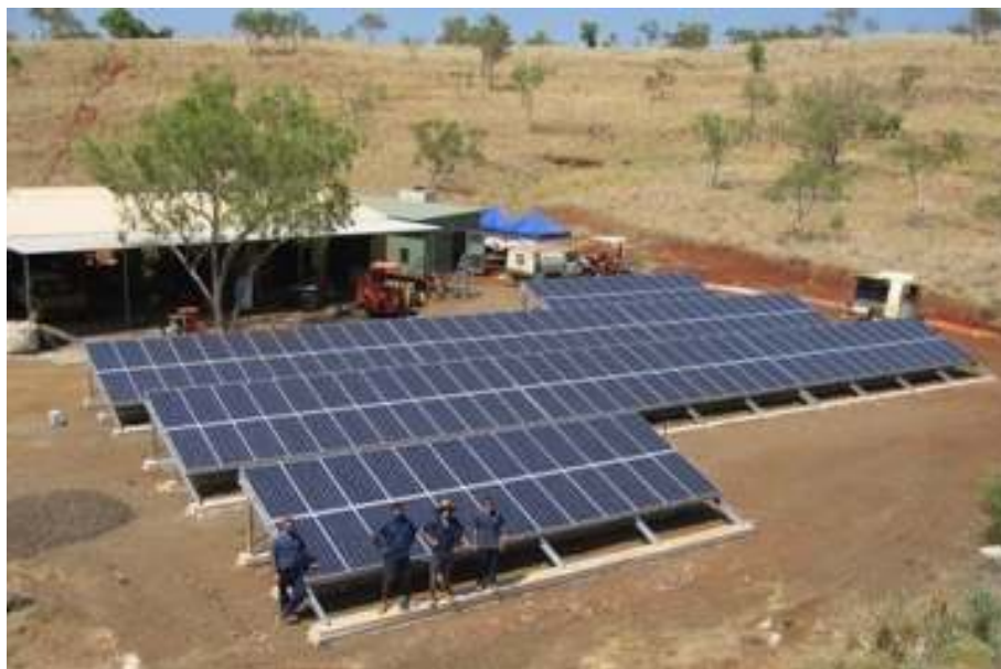
Figure 35. The 192 solar panels of the 32 kW peak power system at the Australian Wildlife Sanctuary Mornington in the Kimberley. The property once used 50,000 L/year of fuel and now uses 7,000 L/year.
