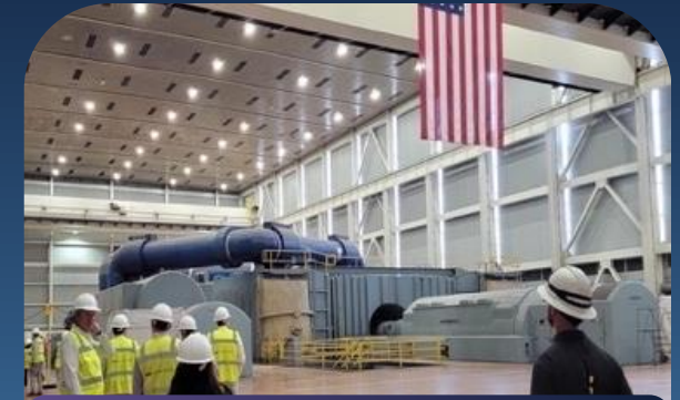
Infinity ONE Prototype and Testing Training Facility
