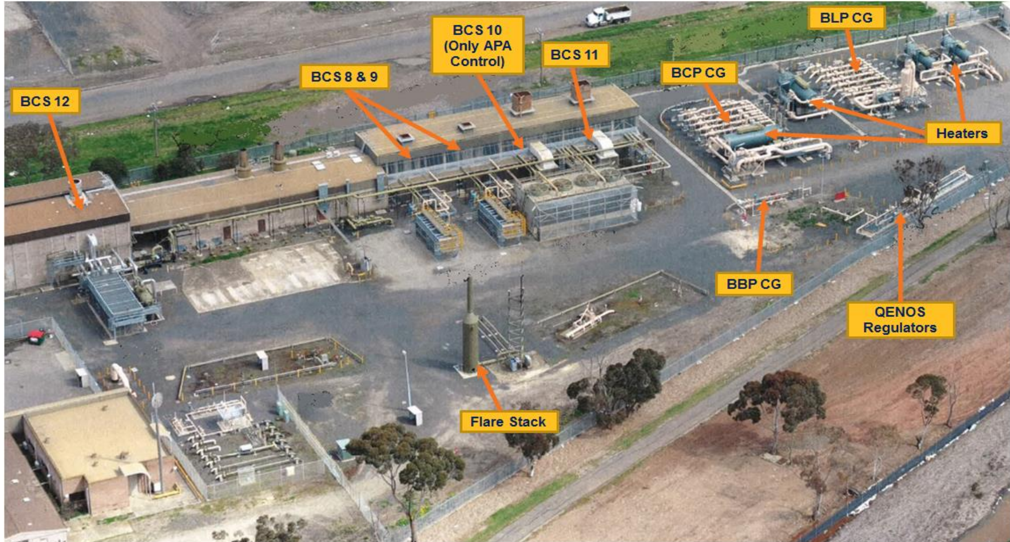
Brooklyn Compressor Station and City Gate, Melbourne western suburbs
