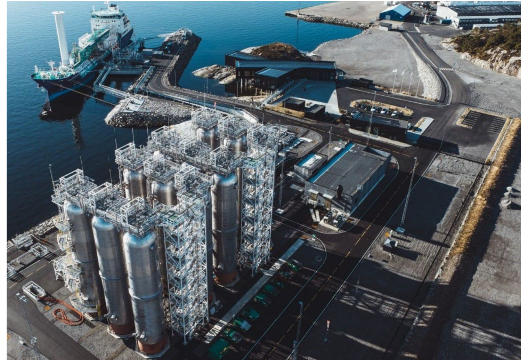
Northern Lights CO 2 receiving terminal in Øygarden, Norway Phase 1 capacity: 1.5 Mtpa. Currently under expansion to 5.0 Mtpa (not shown)
