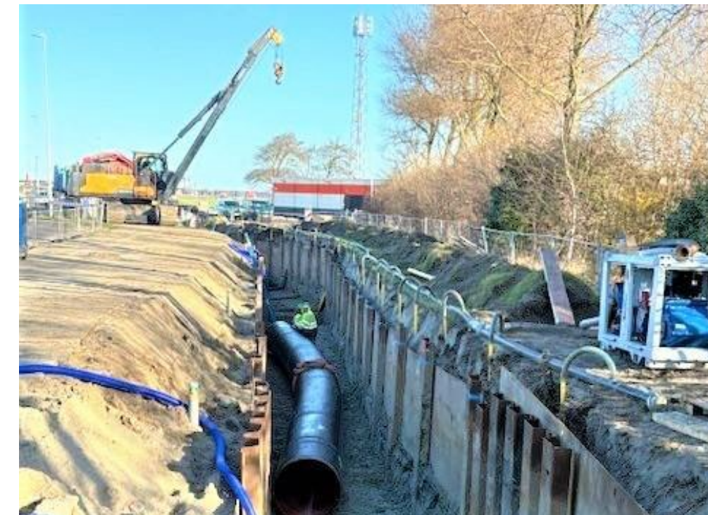
Porthos CO 2 pipeline Network under construction in Rotterdam, Netherlands. Source: European Commission (2025)
