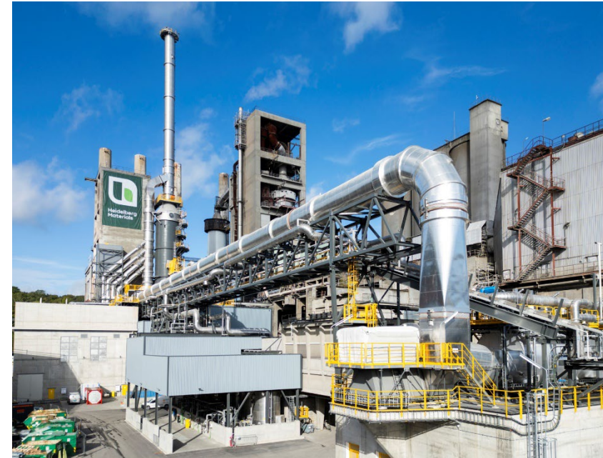
CO 2 capture on cement manufacturing facility. Brevik CCS project, Norway (source: Heidelberg Materials)
